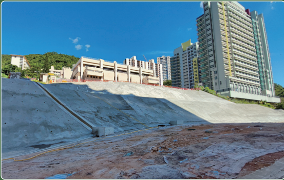
► Demolition of Pokfield Road Residences and site formation works
